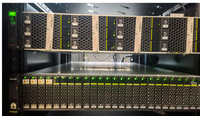
Figure 8: two Huawei optical network controllers (iMaster NCE-T)
